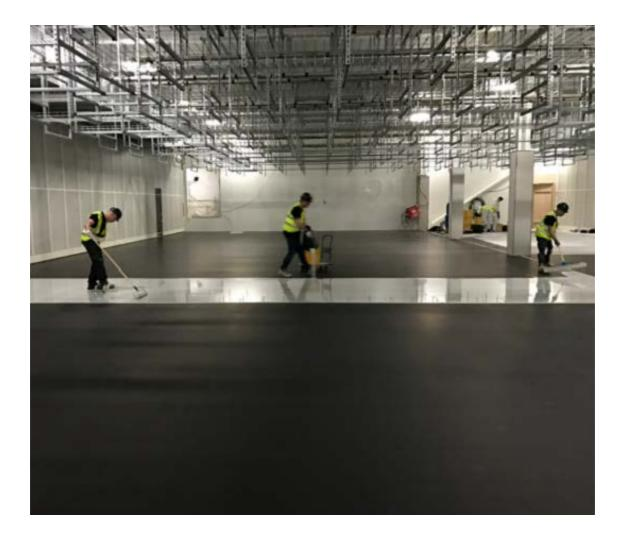
Sika supplied the perfectly-level, anti-static floor system to protect highly-sensitive IT equipment on behalf of one of the world's leading banks. read more
