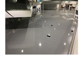
Seamless, anti-static and a perfectly flat floor to precise tolerances were the three essential requirements for this TV studio. The resin flooring system has been installed to the highest specification to ensure the safe movement of cameras and vital equipment.
