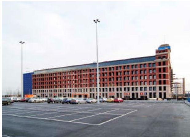
Caption: Massive Refurbishment with Remmers Systems at Fort Dunlop
